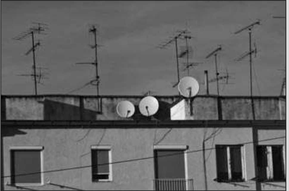
ANTENNAS AND SATELLITE DISHES - There are retrofitted “gardens” of antennas and satellite dishes that cover the tops of buildings all over Zagreb. The wires meander over the sides of the buildings like vines.
