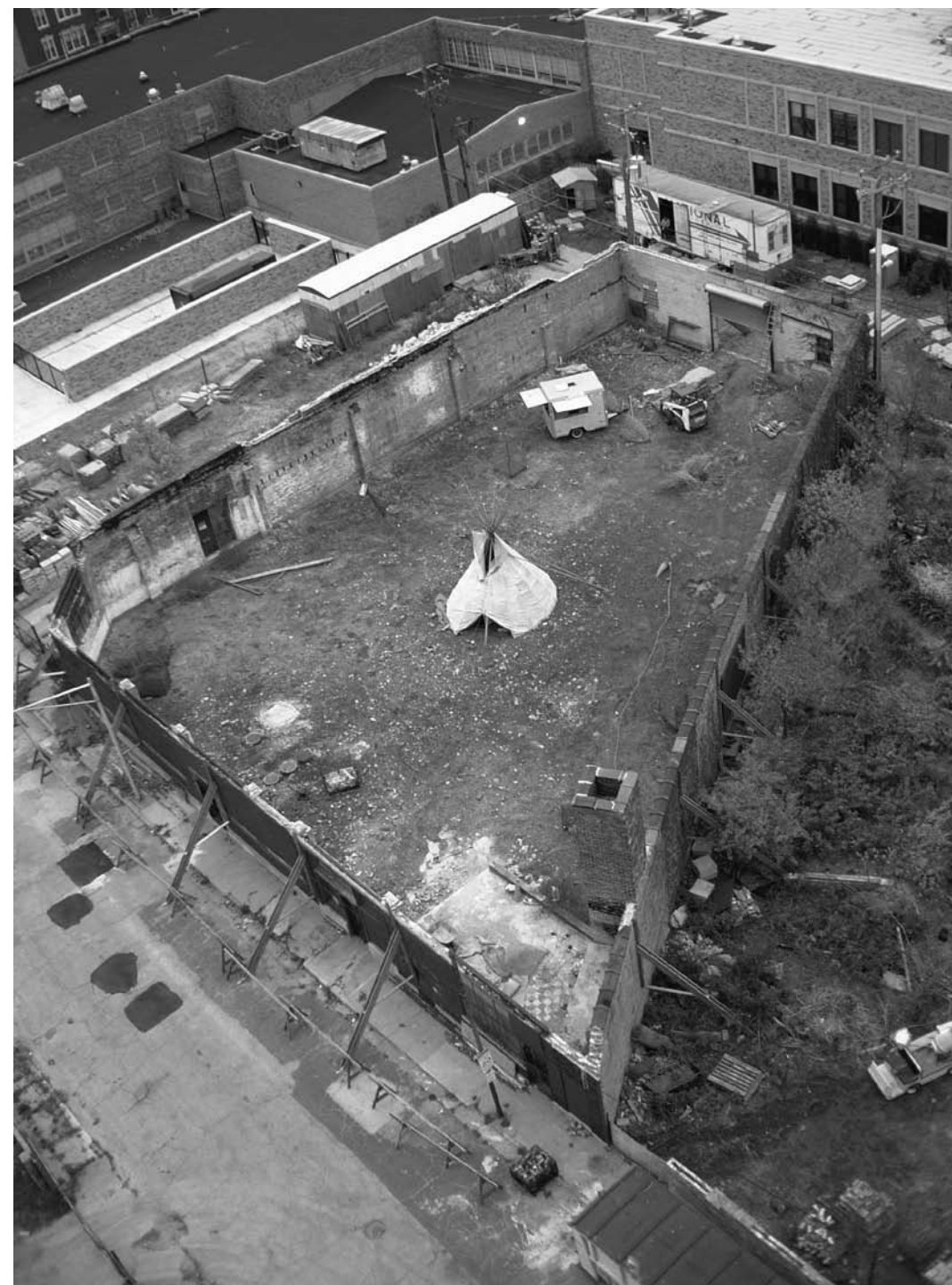
The Experimental Station after the removal of the fire damaged parts of the building, Chicago, photo by Dan Peterman, 2001
