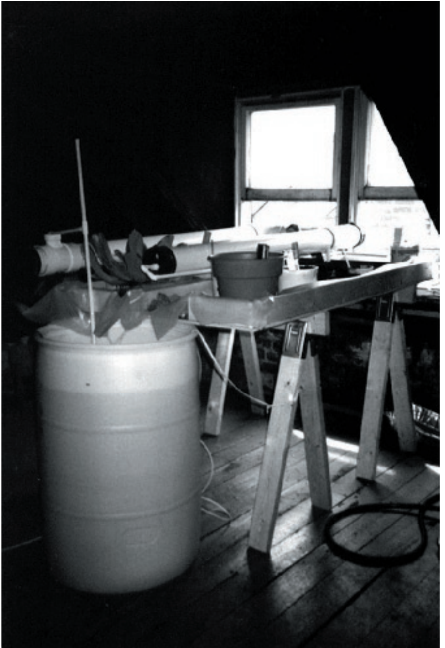
An apartment installation of Eco Vida's Aquaculture system
